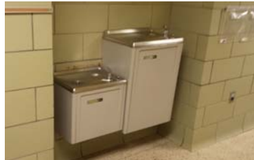
Non-compliant water cooler
