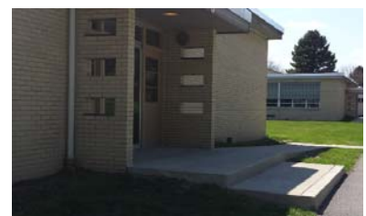
Non accessible – no handrails
