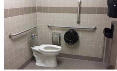
Compliant single user toilet
