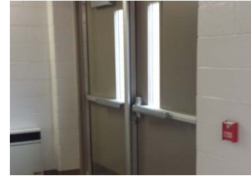
No tactile "EXIT" signage
