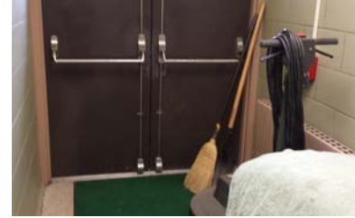
Egress doors blocked
