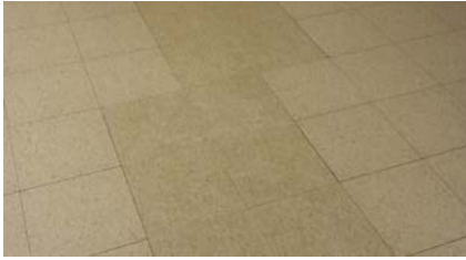
Floor tile patching
