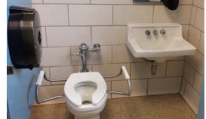
Non-compliant toilet stall
