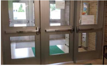
Main egress doors
