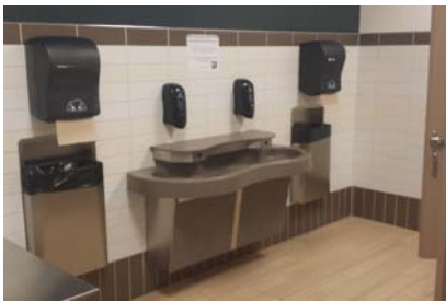
Compliant wash station
