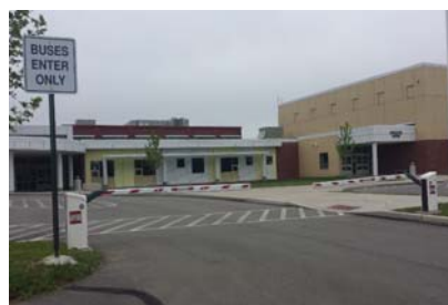
Vehicle Control Point
