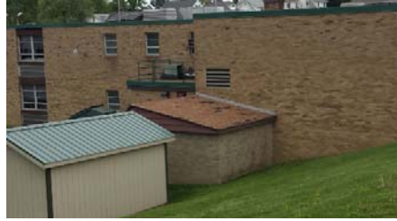
Shingles need replaced
