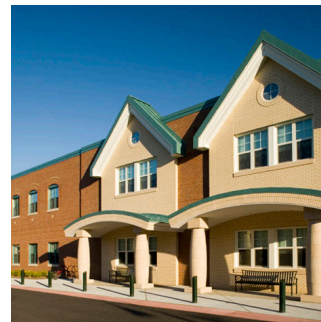
Edgeworth Elementary School Quaker Valley School District Sewickley, PA Additions / Alterations
