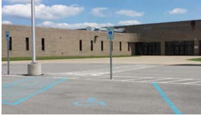
Rear entry accessible route
