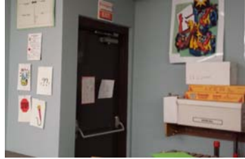
Direct exit from classroom
