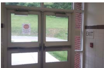
Code Compliant Exit
