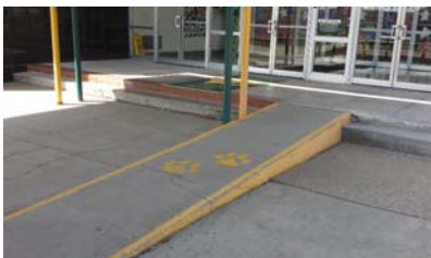
Main entry ramp – no handrails
