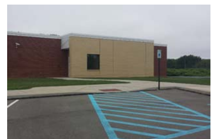
Rear Accessible Entry
