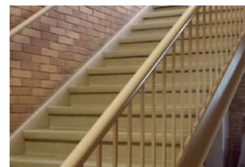
Compliant guards at stair
