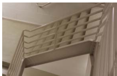
Non-compliant guards at stair
