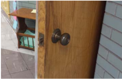
Non accessible door hardware
