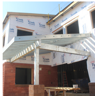
Frazier Elementary/Middle School Frazier School District Perryopolis, PA New Construction
