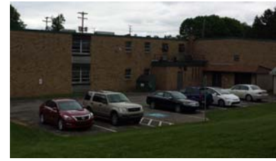
Rear parking area
