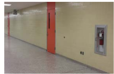
Typical corridor finishes
