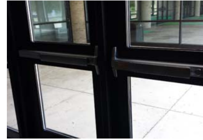
Code compliant panic hardware
