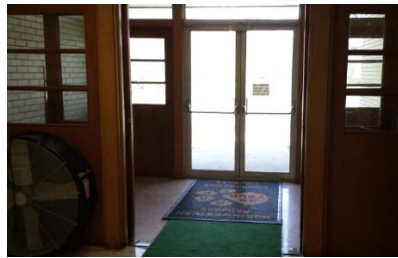
No accessible signage at doors
