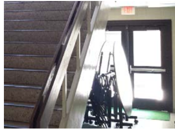
Items stored in stairs
