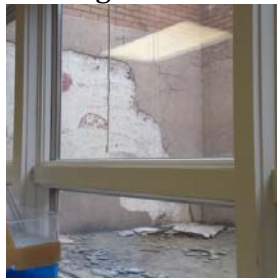
Wall finish delamination
