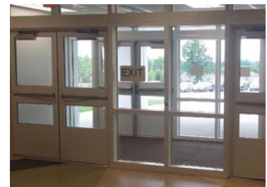
Compliant "EXIT" signage
