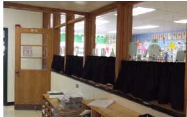
Glazing at Kindergarten
