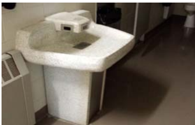
Compliant wash station
